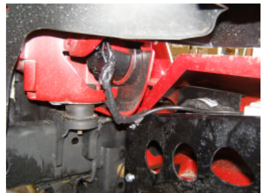
TAPED RHS LOOM
