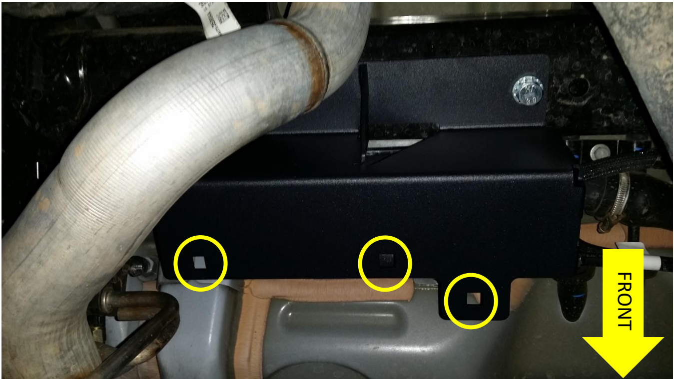
Figure 8 JL-201 Adapter Bracket Bolted in Place
